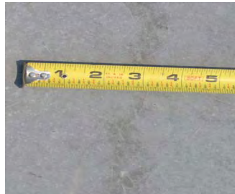
Tight Crack Containment with Fibermesh 650
